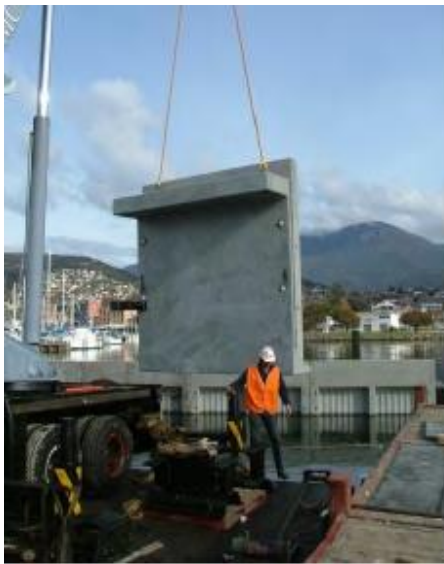
Photo A: Construction of fixed panel wave attenuator – showing fixed panel being lifted into place by floating crane.
