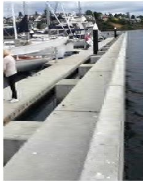
Photo D: View of completed wave attenuator and floating marina.
