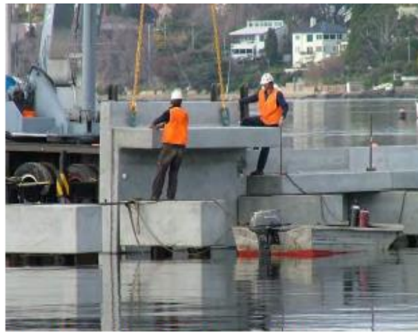
Photo B: Construction of fixed panel wave attenuator – showing fixed panel being positioned onto pile caps
